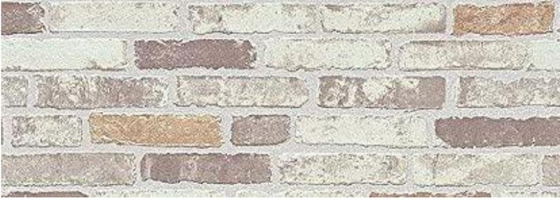
Marmoran Limewash (MLW) coating is a superior decorative coating based on a pure acrylic resin. This limewash is ideal for brick and stone applications for artisan finishes and antique patinas, or for full limewash coverage. When applied correctly, MLW creates a whitewashed brick effect, which can vary depending on the way it is applied and the desired effect.
